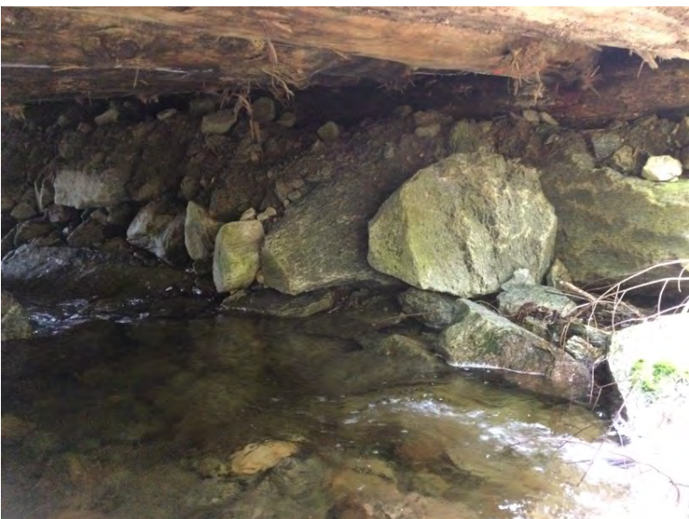
Right Bank Abutment when facing downstream
