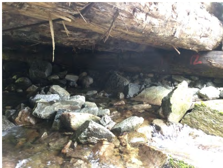
Left Bank Abutment when facing downstream
